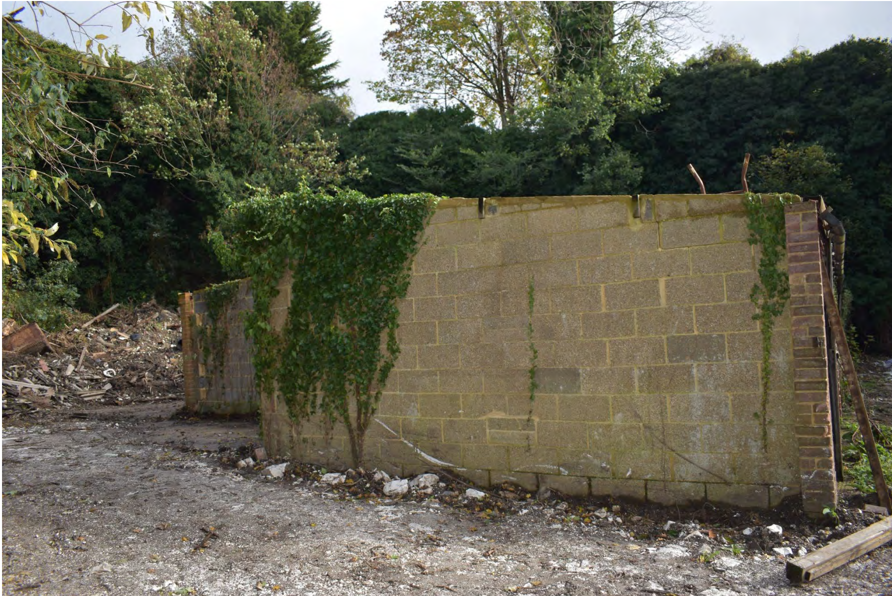
Plate 15: Western end of the garage building (facing)
