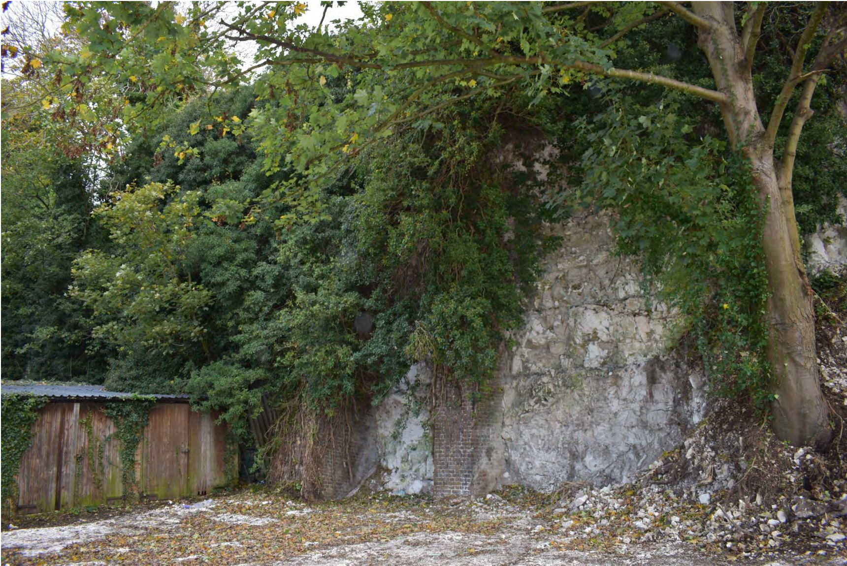
Plate 25: View of the brick buttresses on the eastern side (facing NE)
