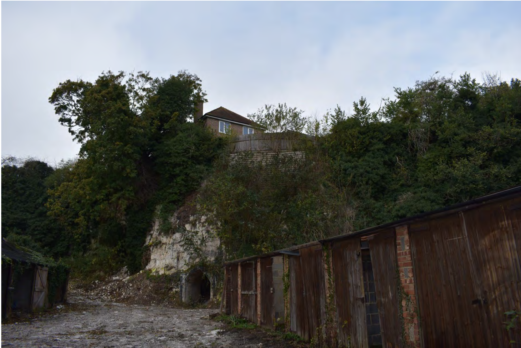
Plate 20: View towards the piled retaining wall to houses above (facing)
